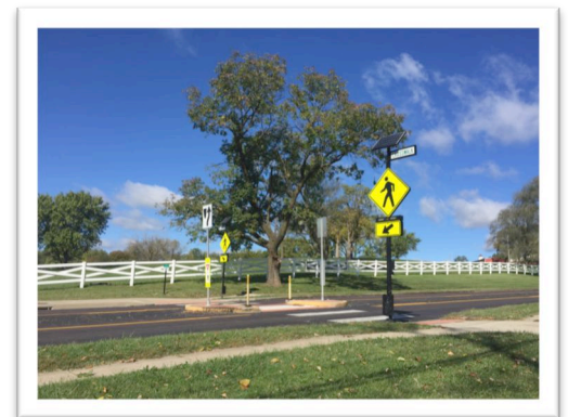
A Rectangular rapid flashing beacon (RRFB)
