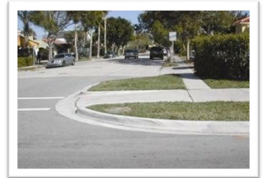
Bulb-out Crosswalk Design. Credit: Federal Highway Administration
