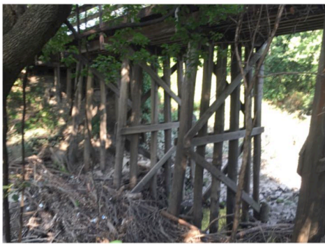
Existing abandoned railroad bridge along Hwy 69 Trail.
